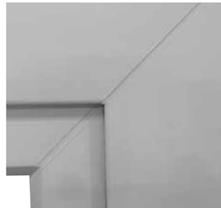
Windows with welded corners (above) are not usually allowed in conservation areas whereas windows with mechanical joints (below) have been approved.
